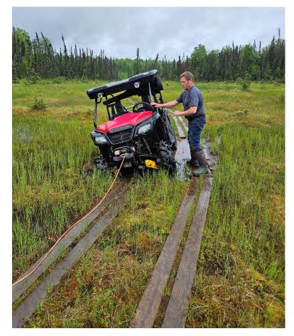
important to conserve the live organic layer on top, so the boardwalk must be constructed very carefully to create a safe place to drive without completely covering and killing the plant life. This means allowing sunlight to reach as much as possible. For this reason, heavy equipment mats are not recommended on floating fen.
